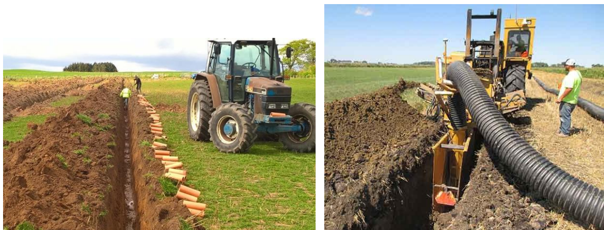
Figure 5. Modern drain installation (Knowlesdrainage.co.uk)
